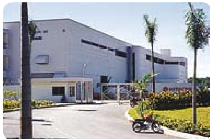
Hitachi Air Conditioning Products (M) HAPM works, Malaysia
