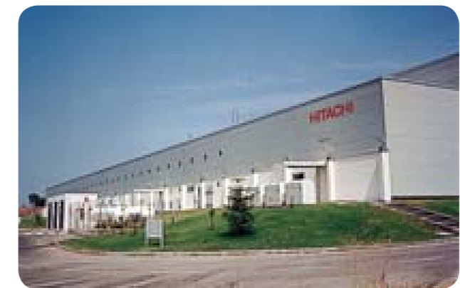
HITACHI Air Conditioning Products Europe HAPE Works, Spain.
